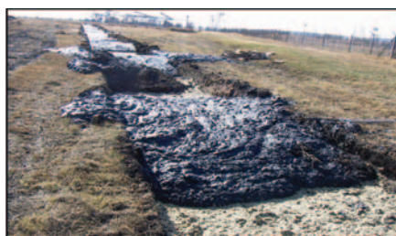
Moved to Treatment Area
